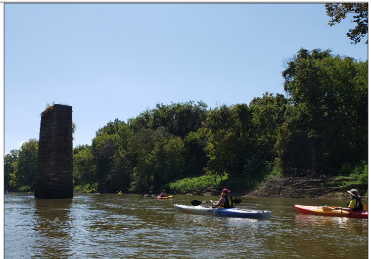
This trestle carried the narrow-gauged Milton & Sutherlin line -- built to connect Milton with the Danville-Richmond line -- across the river.
