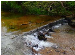
Blackberry Creek after the repair
